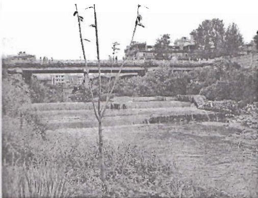
Figure 2.3: Bed Armoring using the concrete floor in Balkhu Bridge Kathmandu.
